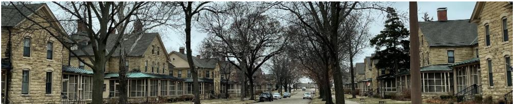
Figure 5.b: Historic housing on Fort Riley is a local example of how the consistent application of design elements provides character cohesion
