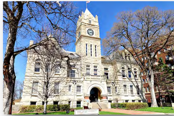
Figure 14 Riley County courthouse.
