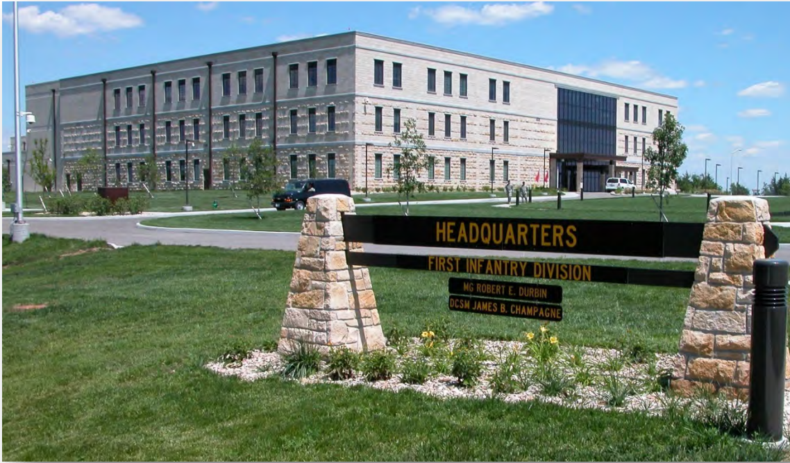
Figure 30 Fort Riley Headquarters
