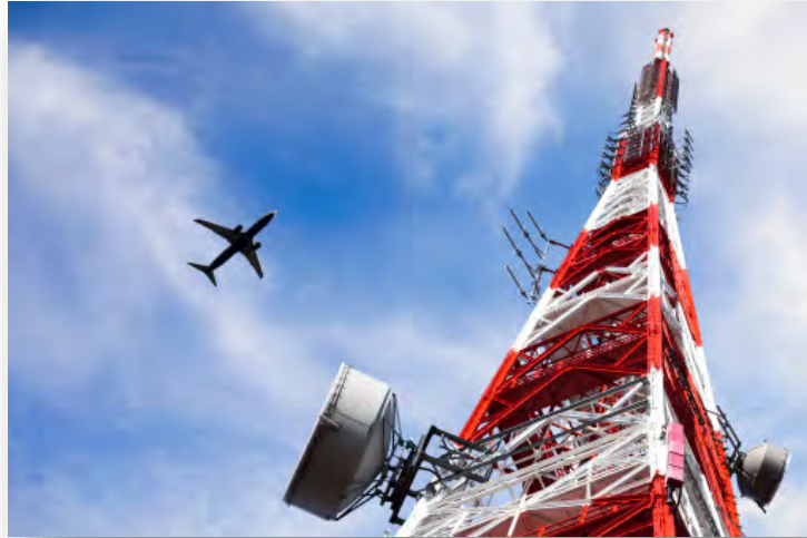
Figure 40 Telecommunication towers can interfere with the safe navigation of airplanes if proper regulations aren't in place
