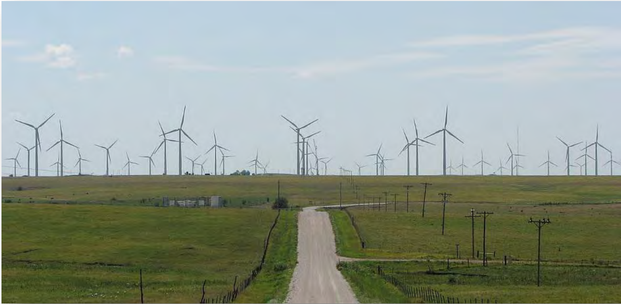
Figure 55 The moving blades of a wind turbine create a Doppler effect that can create communication interference
