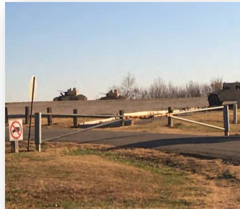
Figure 60 Approximately 22 miles (28%) of the 78 miles of Fort Riley's perimeter is fenced.
