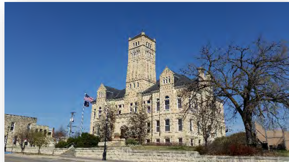
Figure 12 Geary County courthouse.
